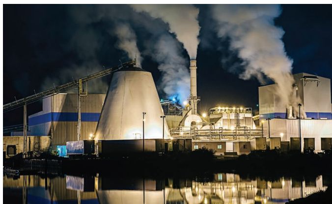
Emissions from this mill in Port Angeles, WA, were subject to the Cluster Rule.
